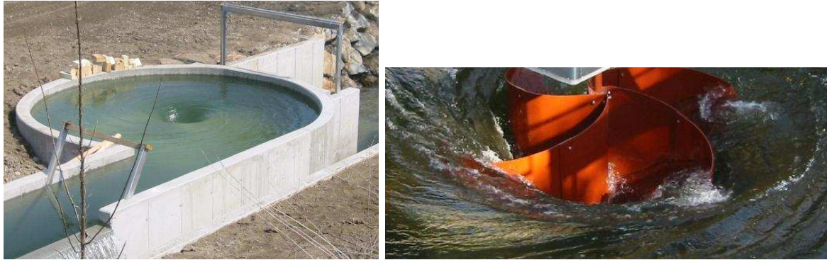
Inlet with overflow and vortex basin during construction - Image: zotloeterer.com .
